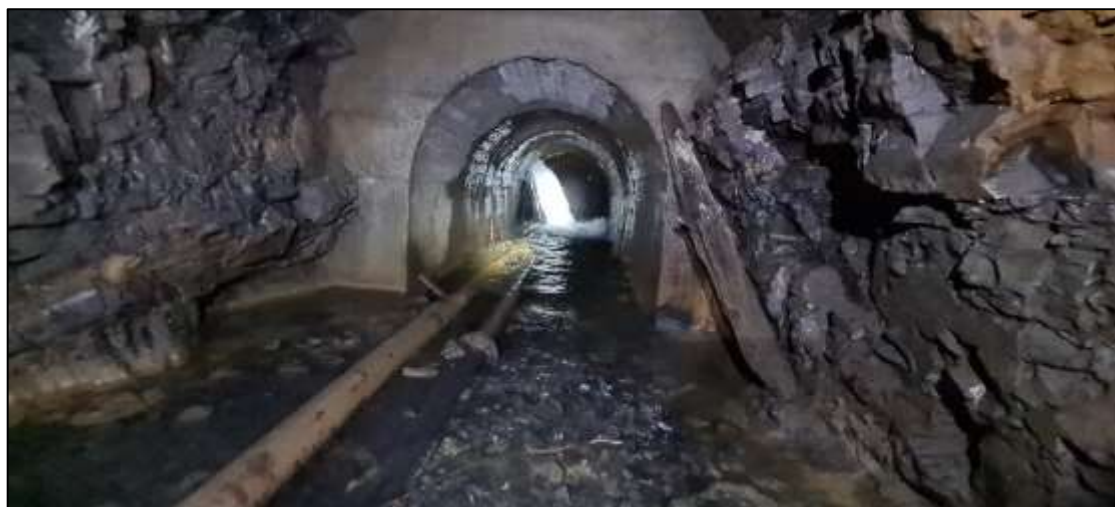
Figure 18-14. Underground Drainage Gallery
