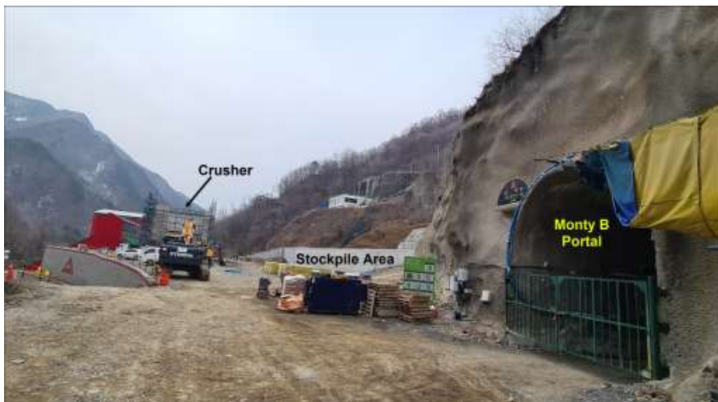
Figure 18-4. ROM Stockpile Area Next to Monty-B Portal.
