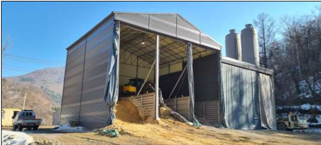
Figure 18-5. Surface Batch Plant
