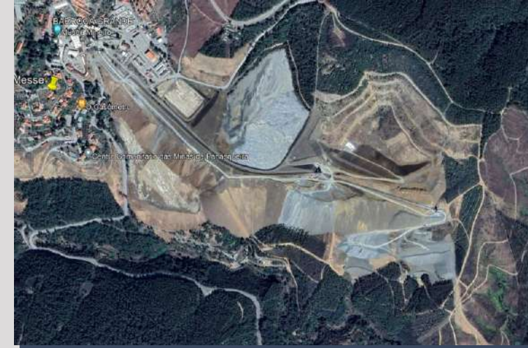
In-house completed & designed new fine tailings pond (on the right) – Capacity for a further 27 years
