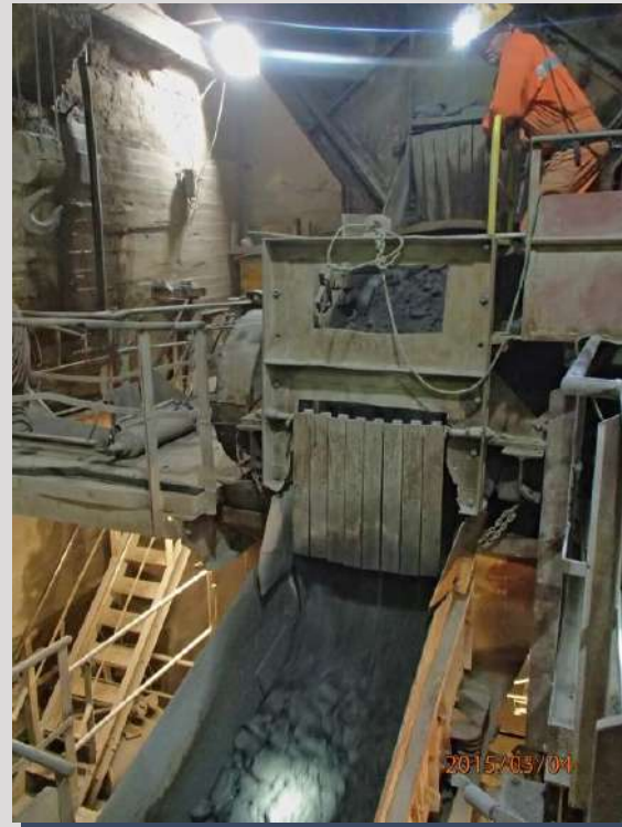
Underground crushing chamber
