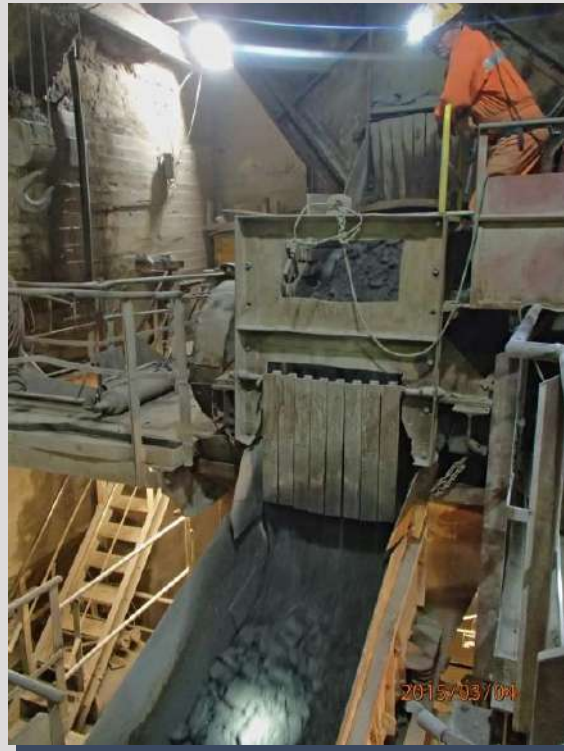
Underground crushing chamber
