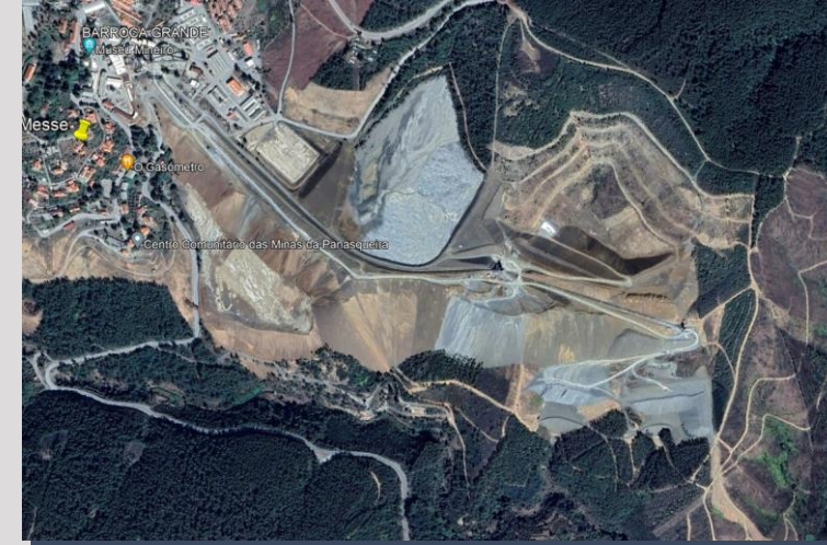
In-house completed & designed new fine tailings pond (on the right) – Capacity for a further 27 years
