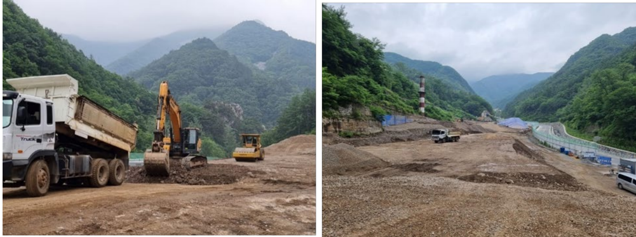
Photo of Scalping Work Site
