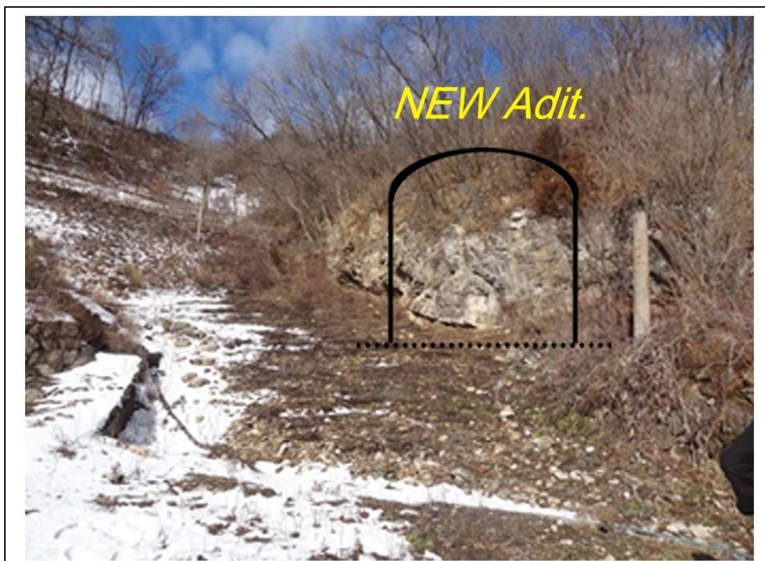
Figure 16-38. New Adit Portal Position, For -1 Level
