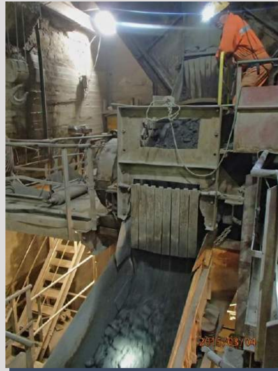
Underground crushing chamber
